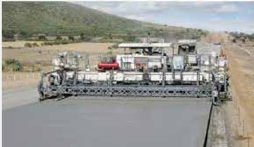
Image 4: Concrete paver roads
