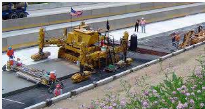
Image 5: Concrete paver roads
