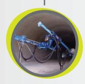
Ec0mine forms a thixotropic paste that is sprayed onto the prepared rock face.
